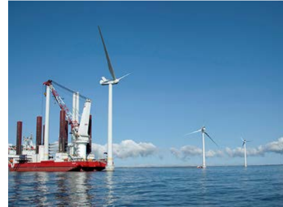
2015 Luchterduinen project (Netherlands) V112-3.0MW x 43WTGs 2 WTGs/1day
